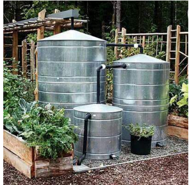
Example Rainwater Collection System
