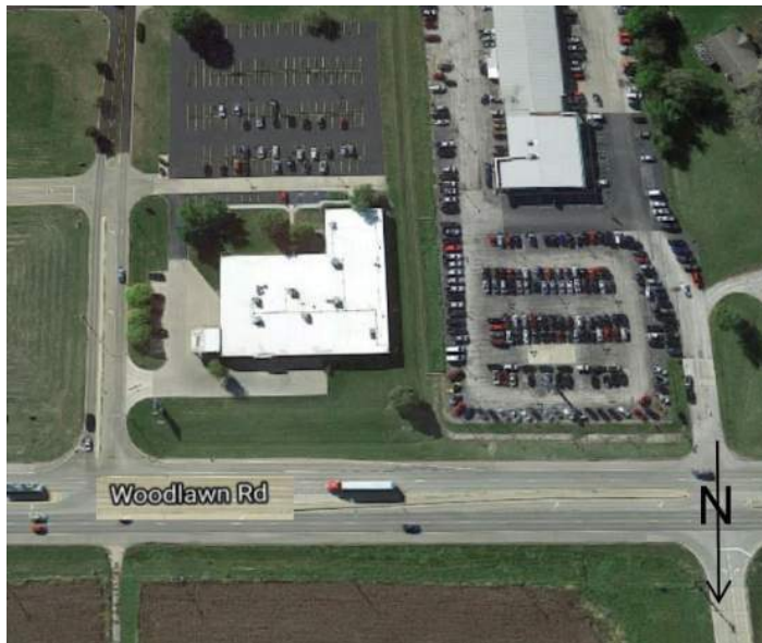
Lincoln Campus Aerial View
