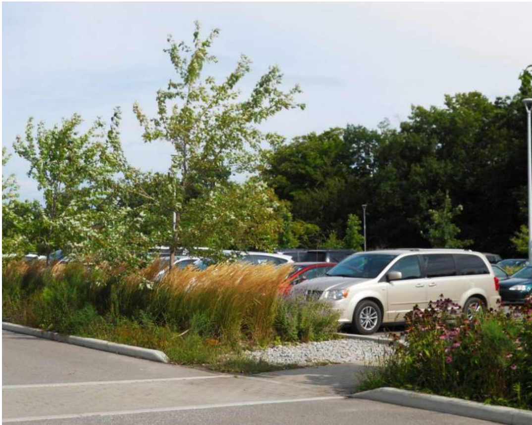
Typical Bioswale within a Parking Area
