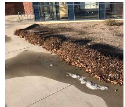
Existing Landscape Maintenance Issues
