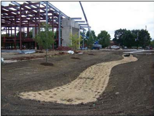
Vegetative swale preparation
