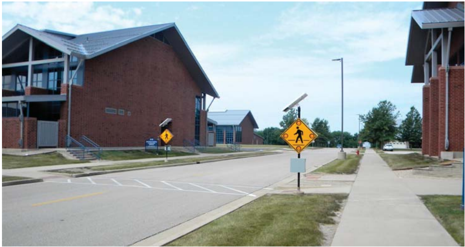
Looking west at crosswalk between ICN and WDC
