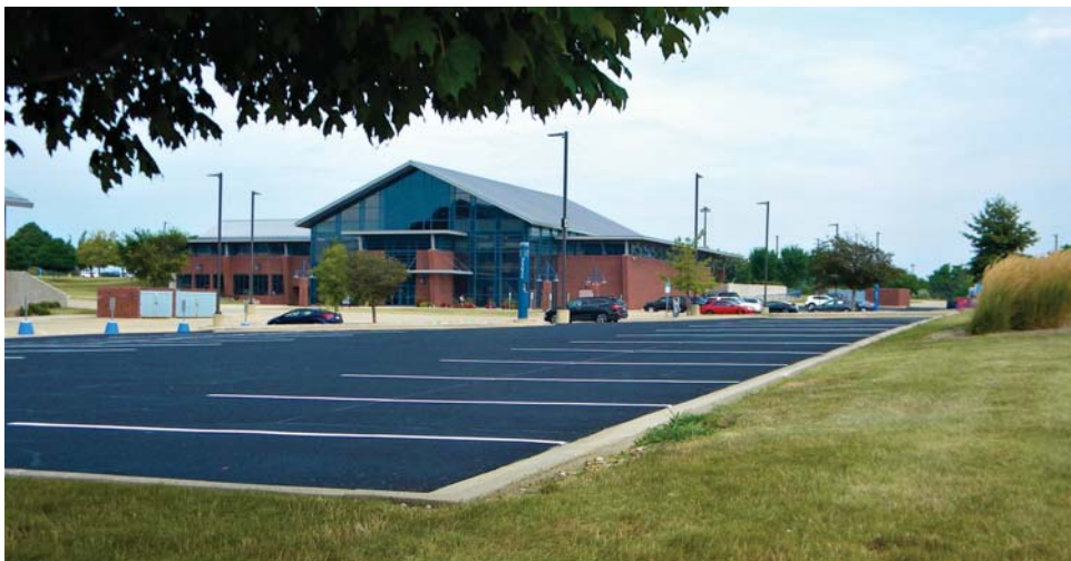
Looking north at parking with FRC and Fitness/Recreation area
