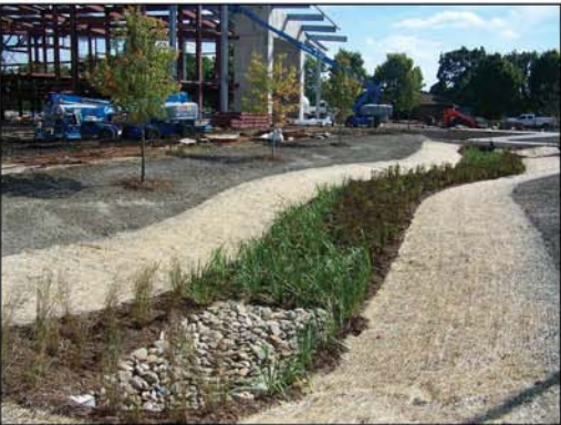
Vegetative swale planting
