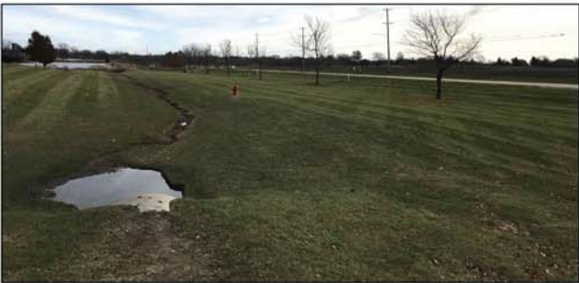
Drainage swale south of Normal Readiness Center
