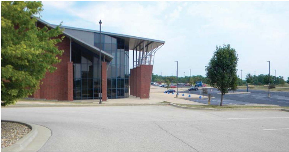
Looking north at CEC
