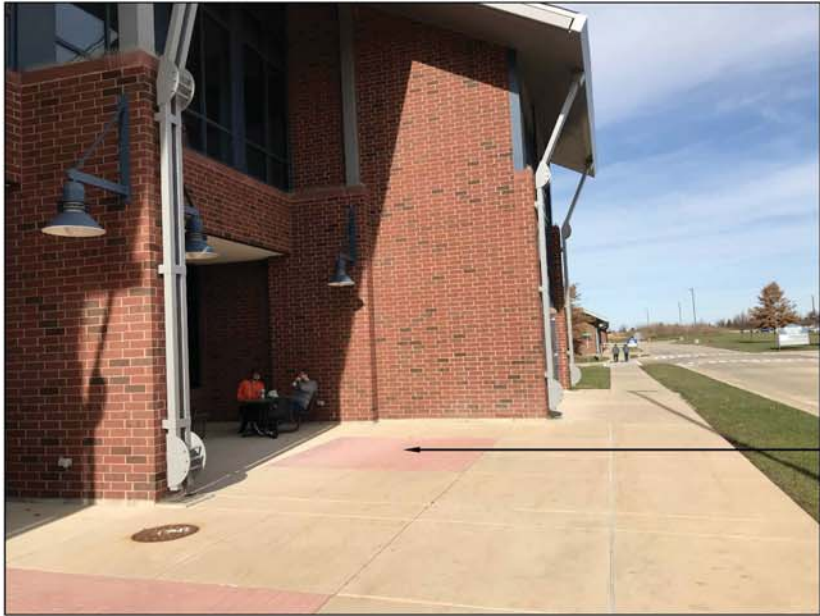
Existing tinted concrete to be removed, soil excavated and replaced, and trees and groundcover installed
