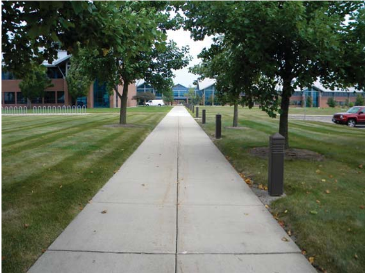
Looking north along sidewalk
